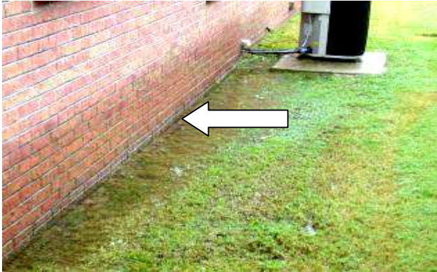
A view of water concentration around the back left exterior. A view of water penetration inside the garage.
