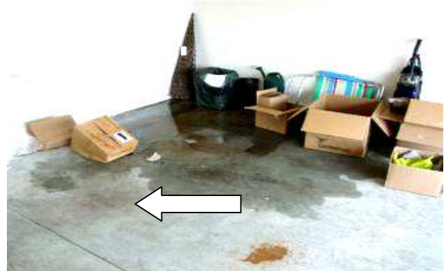
A view of water concentration around the back left exterior. A view of water penetration inside the garage.
