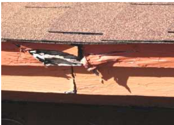
A view of deteriorated fascia board along the front side of the house.
