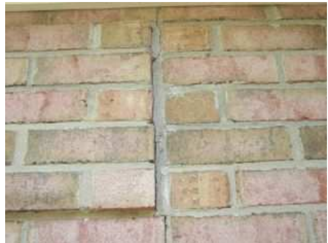
A view of small exterior settlement cracks along the front side.
