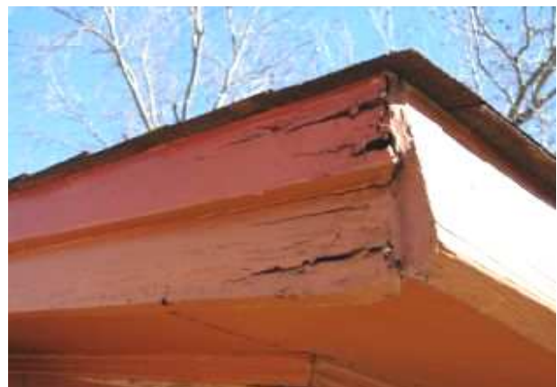
A view of deteriorated fascia board along the front side of the house.
