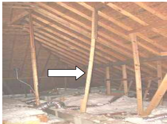
A sample view of bent center post located inside the attic space.
