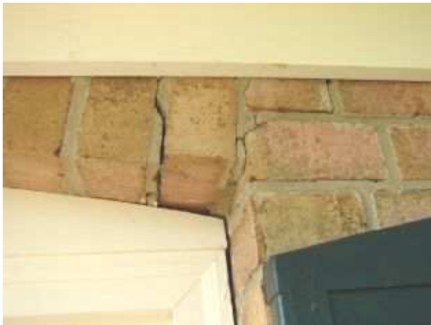
A view of small exterior settlement cracks along the front side.
