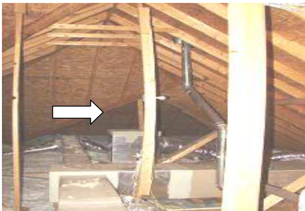
A sample view of bent center post located inside the attic space.
